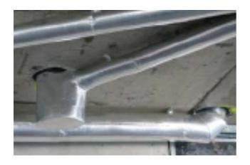
Improved vibration damping with microcellular noise barrier and solid foam barrier
